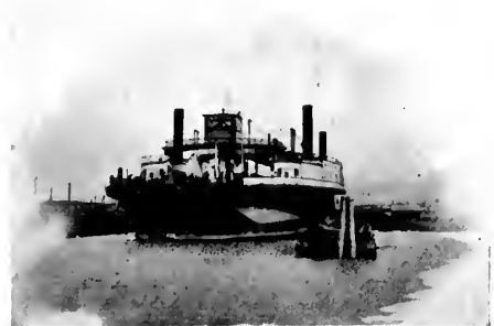
The 5,000-ton Crandall marine railway at the Southern Pacific Shipyards, East Oakland, California. The "Contra Costa," the largest car ferry in the world and the largest wooden craft ever built, is shown on the dock.
